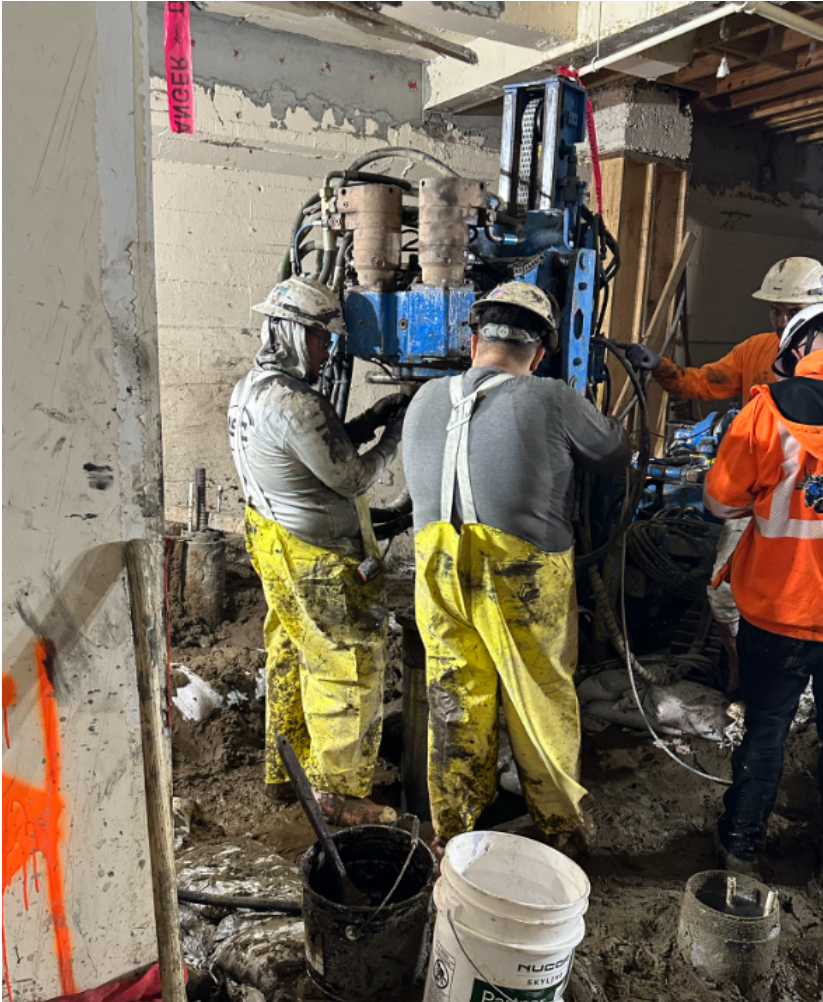
2/5: Tower crane micro pile drilling
