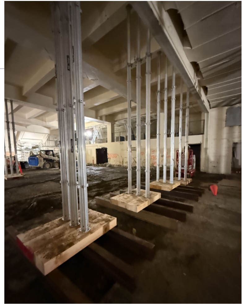
2/14: Deck support installed for structural demolition
