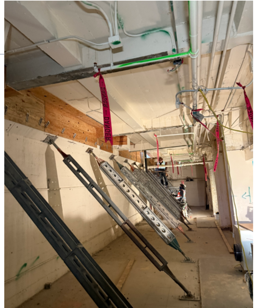
Temporary shoring during the installation and curing of the waler beam
