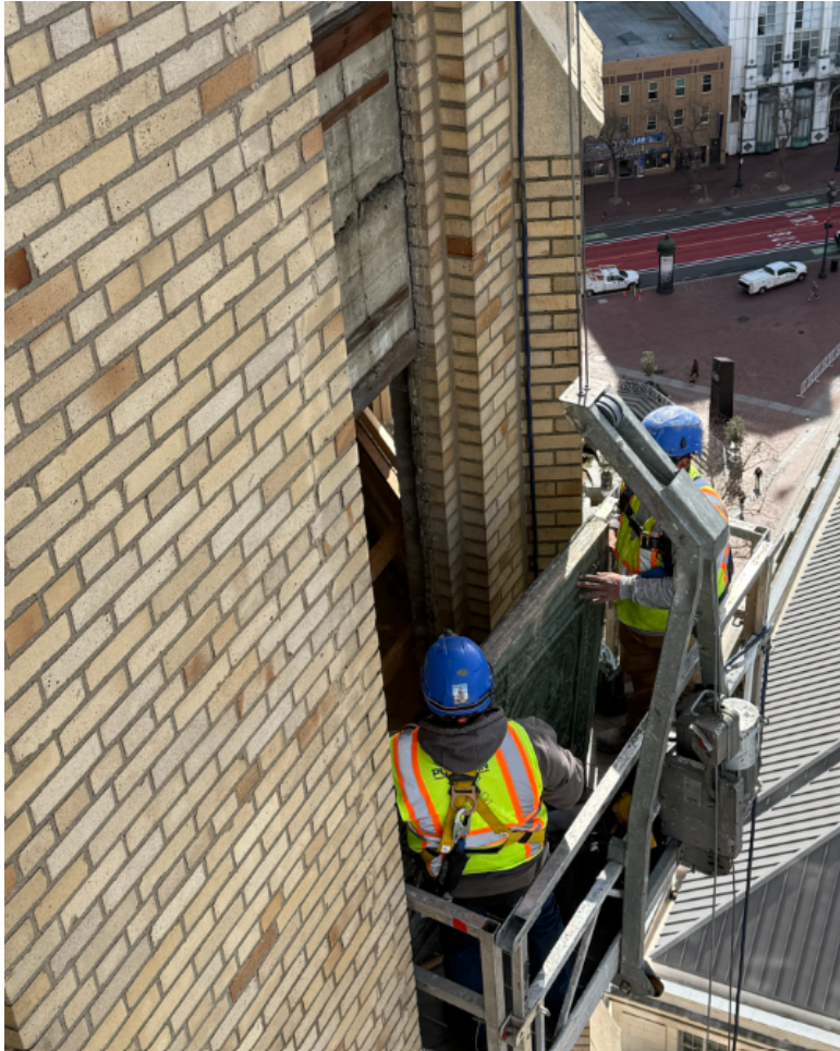
2/18: Exterior copper panel removal for tower crane tie-in
