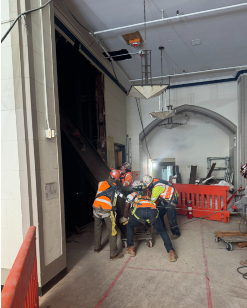
1/15: Hoisting steel beam through elevator shaft for installation
