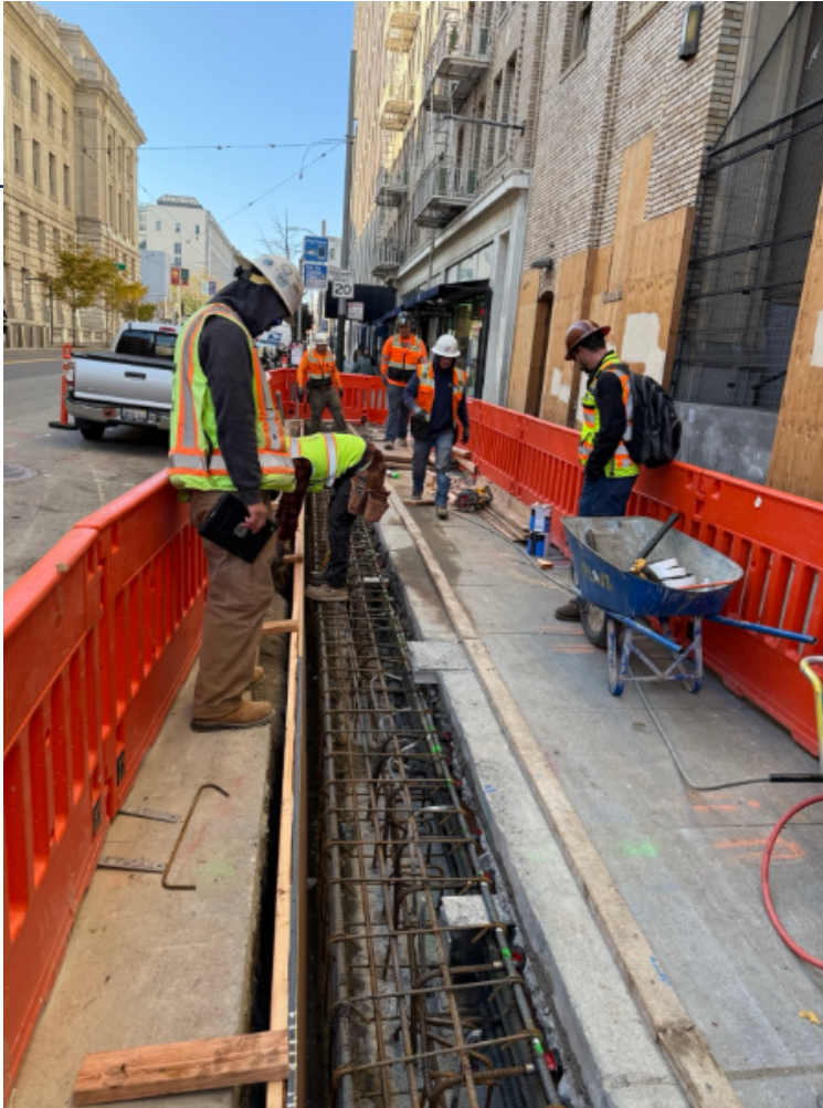
Installation of the waler beam along McAllister
