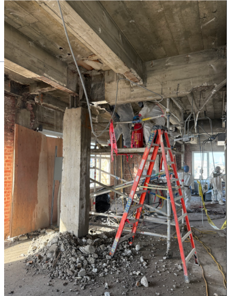
Abatement and demolition to be ready for the steel installation
