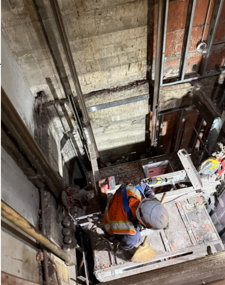
2/12: Complete remaining elevator cab demolition
