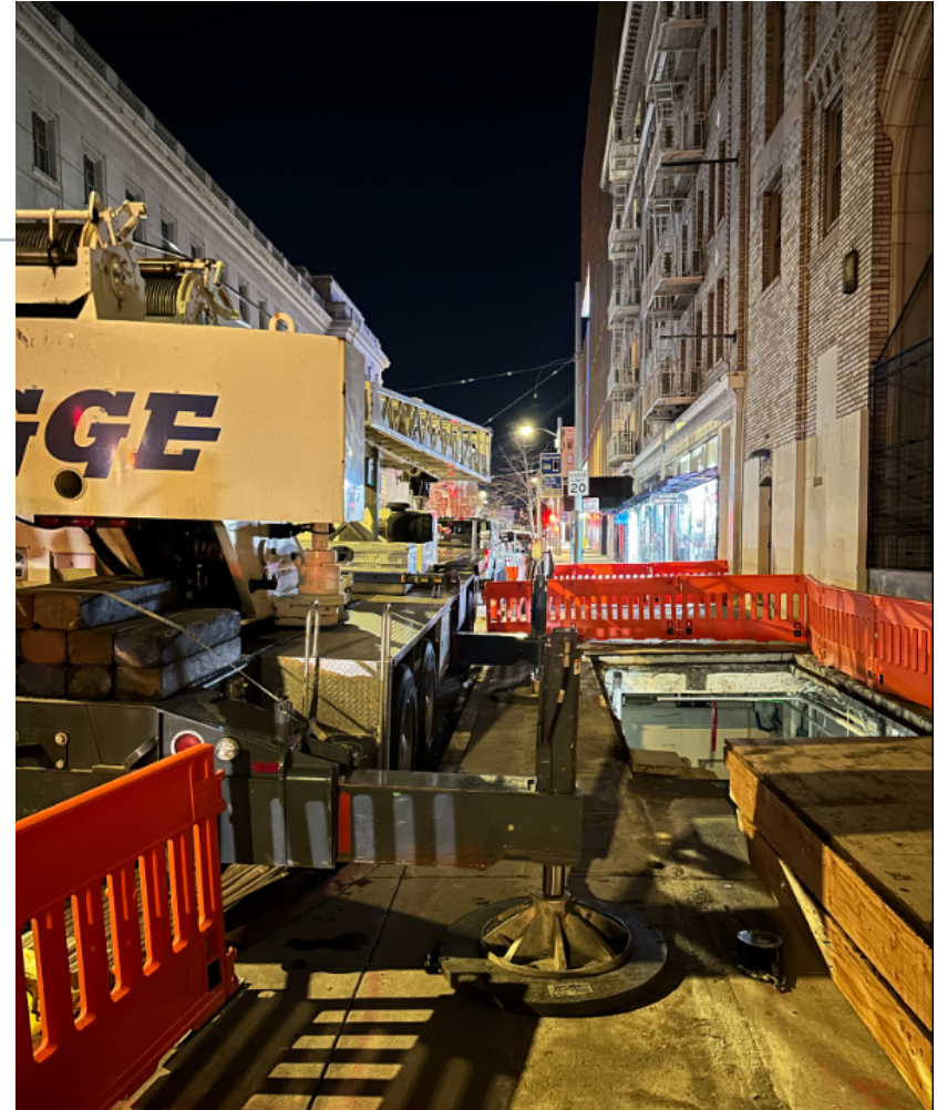
2/8: Equipment off-haul after micro pile installation
