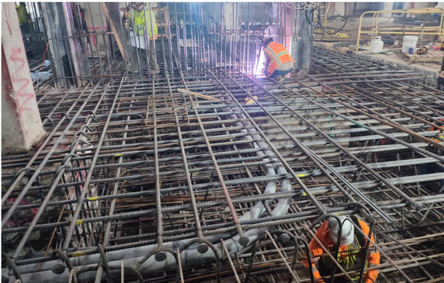
Top Rebar Installation -2025.12
