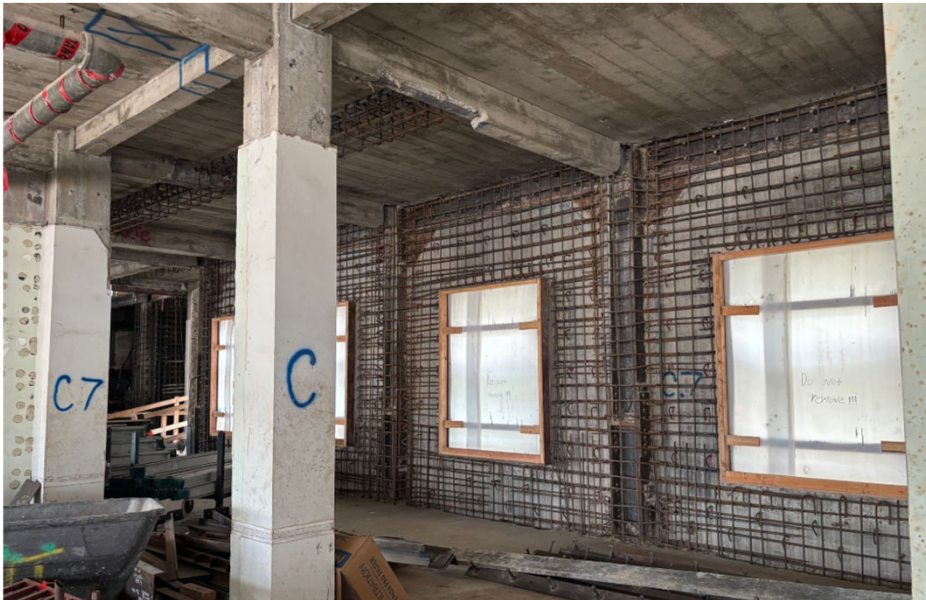
New Concrete Overlay Wall
