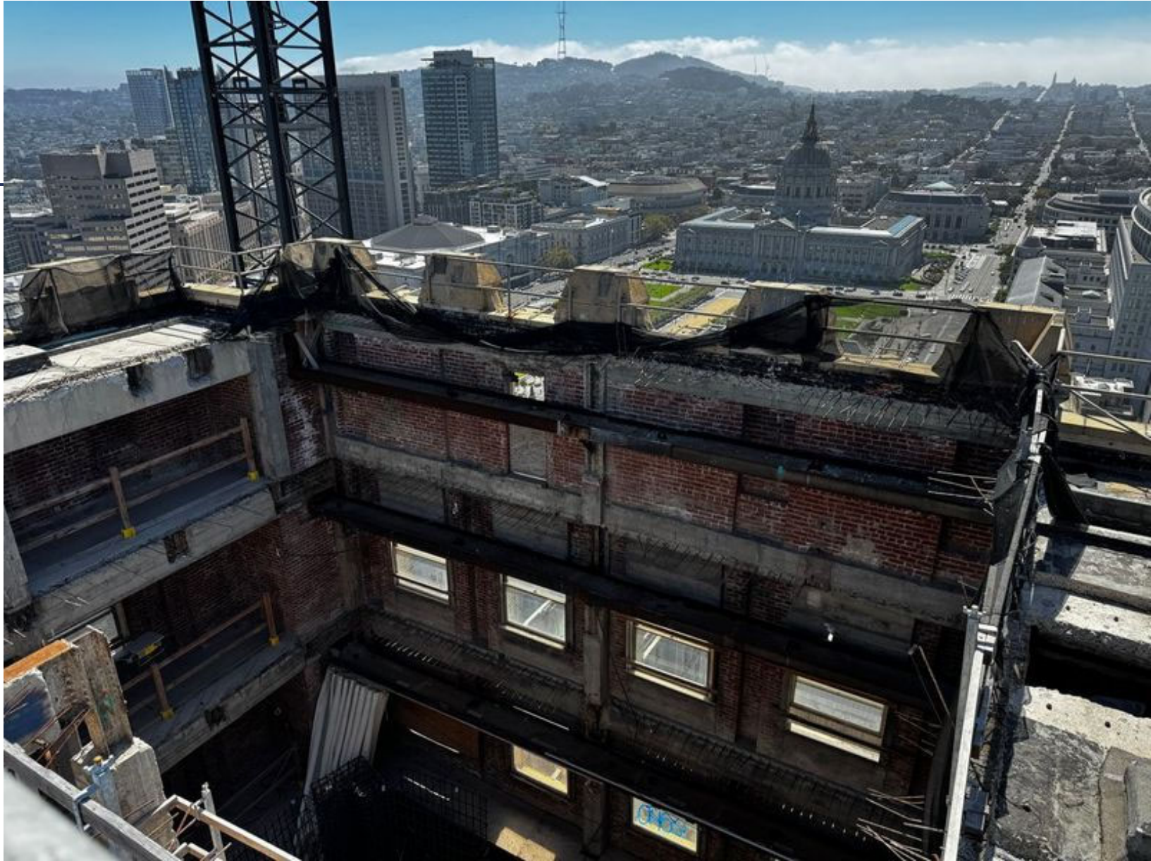
New Building Core
