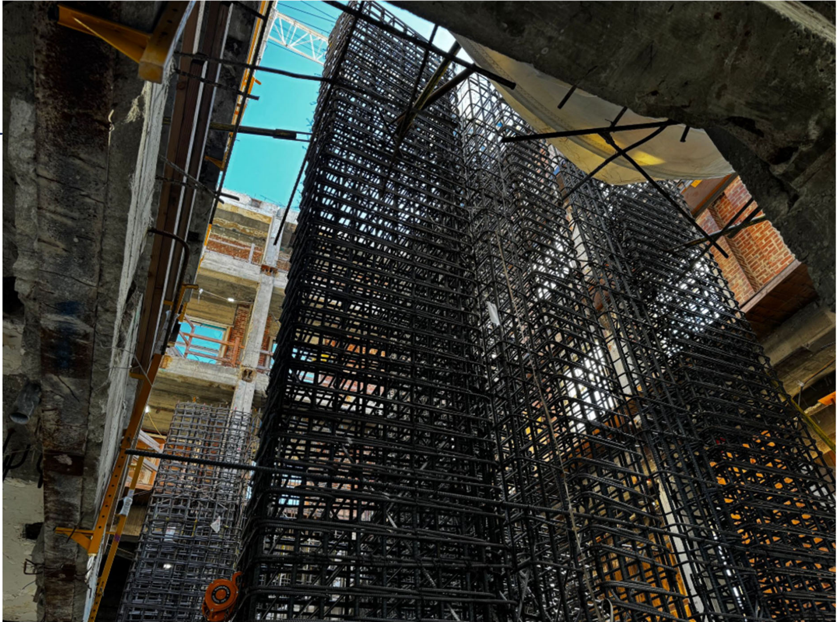
New Building Core
